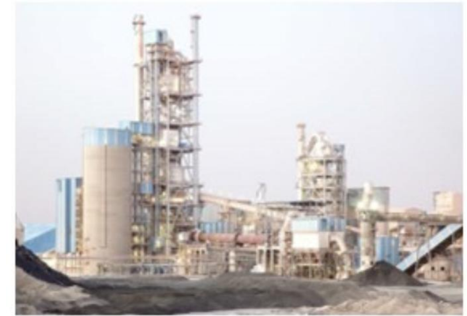
Digital solutions that integrate data and real-time optimisation of processes throughout a cement plant can help boost productivity and reduce unplanned downtime.
